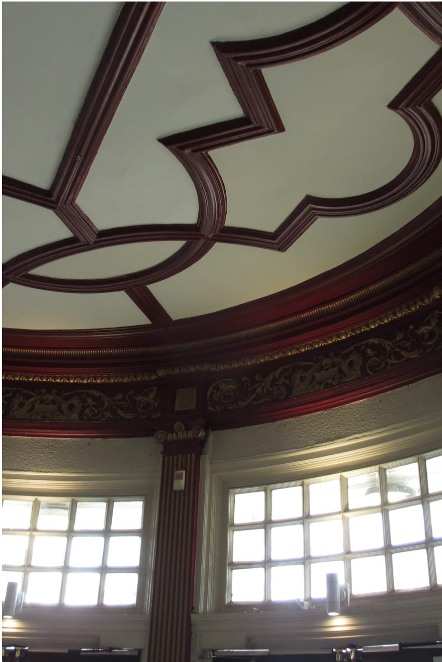
Gate Cinema W11
